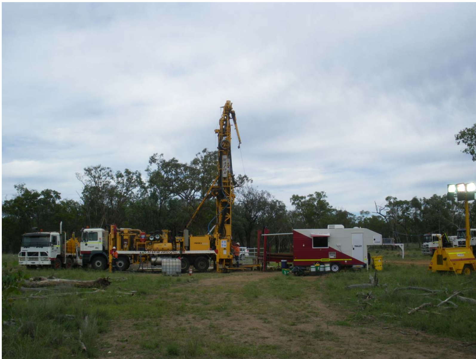
Figure 3: Working Rig – EPC 1623
