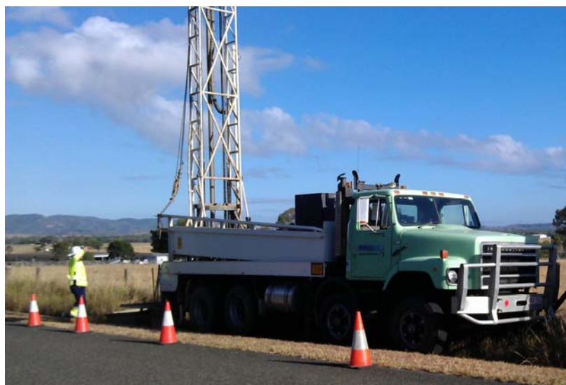
Figure 2: Drill Rig on Site EPC 2239.
